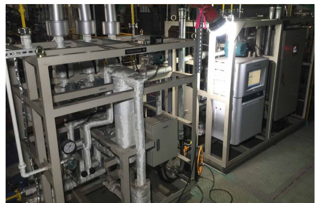
Figure 6 External view of stations
