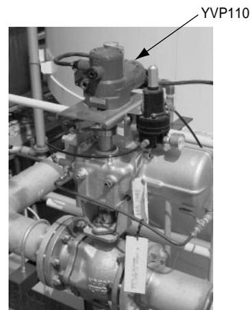
**Figure 1** YVP110 Installed in Actual Plant
