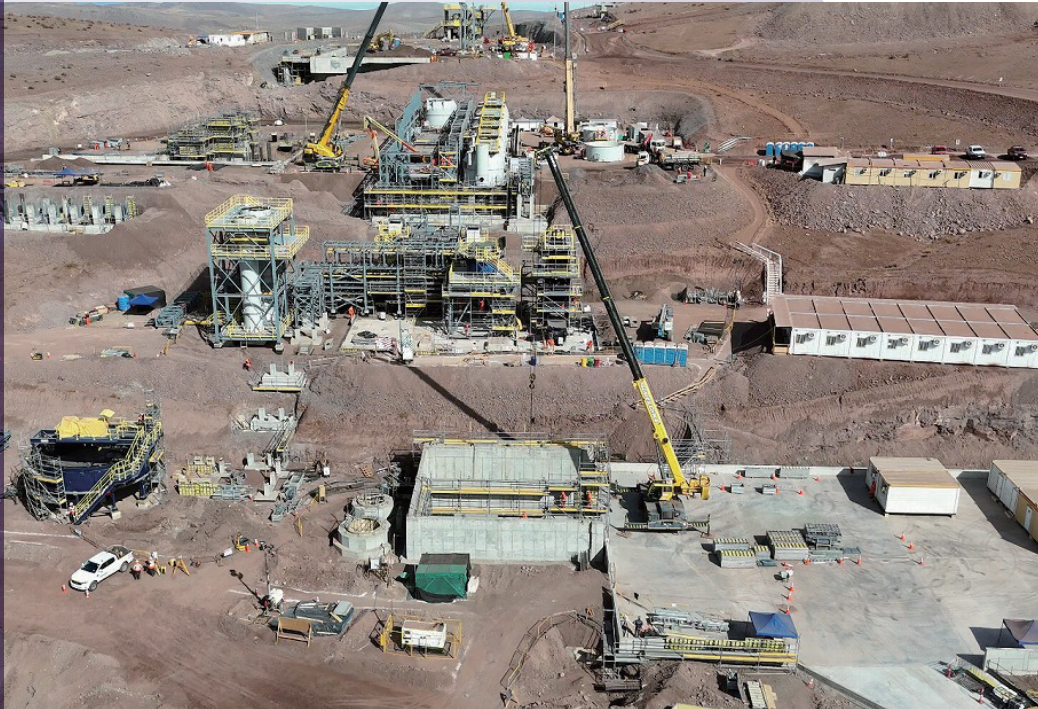
Minera Arqueros plant under construction, May 2025
