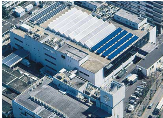
Photovoltaic Power Generation System
