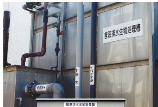
Bio-treatment Facility (at Headquarters)
