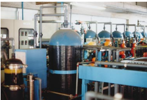
Wastewater Treatment Facility (at Headquarters)
