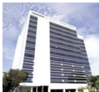
Yokogawa Engineering Asia Pte Ltd (YEA) Yokogawa Electric Asia Pte Ltd
