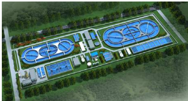
Industrial wastewater treatment facility (Jiangsu, China)
