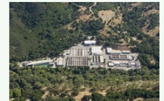
The Tapia Water Reclamation Facility situated in the suburb of Los Angeles, California
