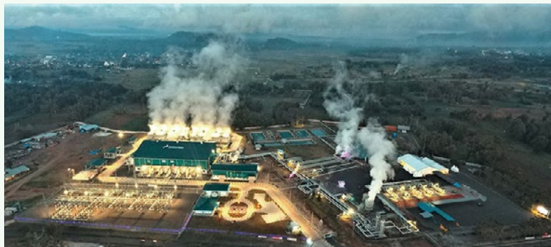
The Lahendong geothermal power plant
