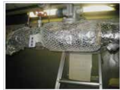
Additional insulation on pipes
