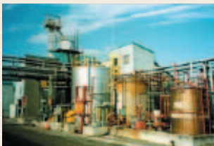
External view of plant
