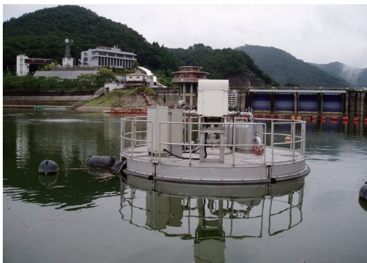
Installation of the system at the Kamafusa Dam Reservoir
