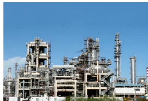
A plant that uses Yokogawa's industrial automation control technology
