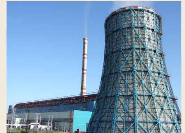
Thermal Power Plant No. 4 in Ulaanbaatar
