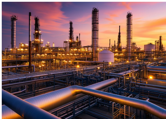
Pipelines showcasing industrial energy production
