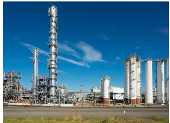
Figure 1 - Refinery Distillation Column
