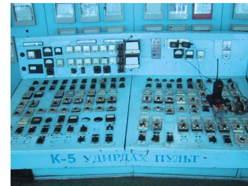
Original boiler control panel
