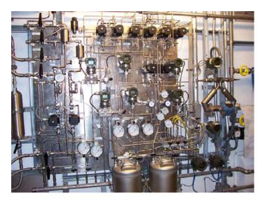
Figure 4. This sampling system for an anlyzer installed in a petroleum refinery provides an idea of the complexity of measuring the critical attributes of gasoline.
