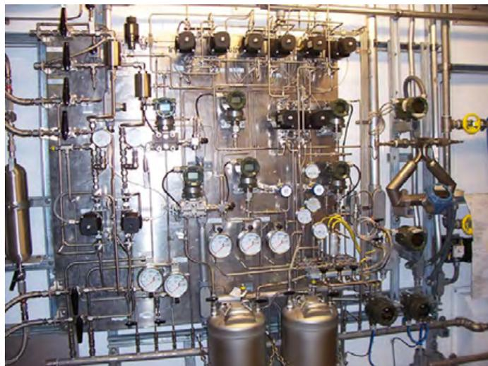
**Figure 4.** This sampling system for an analyzer installed in a petroleum refinery provides an idea of the complexity of measuring the critical attributes of gasoline.
