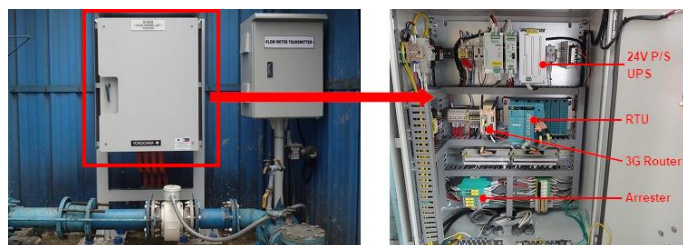
Monitoring box at pumping station
