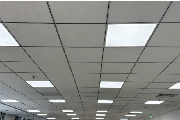
Switching to Energy-Efficient Lighting
