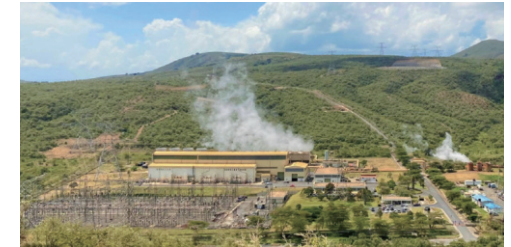
Olkaria II Power Station
