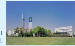
Yokogawa Electric China Co., Ltd.
