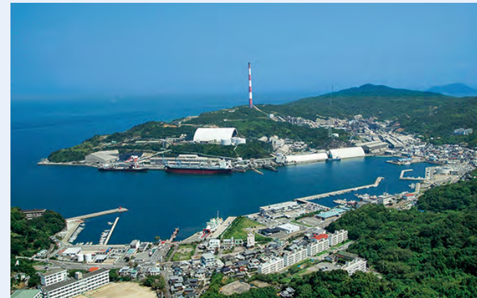
JX Metals Smelting Co., Ltd. Saganoseki Smelter & Refinery
