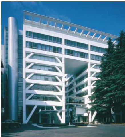
Energy-efficient, New Head Office Building
