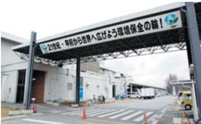
Truck Loading and Unloading Zone (YMF Kofu factory)
