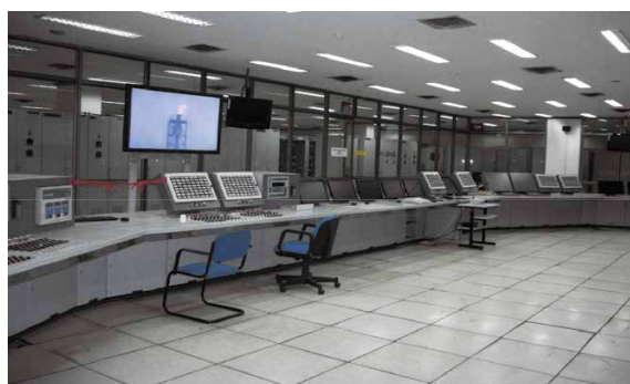
Before and after revamp photos of the central control room (CCR). The CCR layout was jointly designed by IOCL and Yokogawa India. The number of consoles was increased to improve efficiency.
