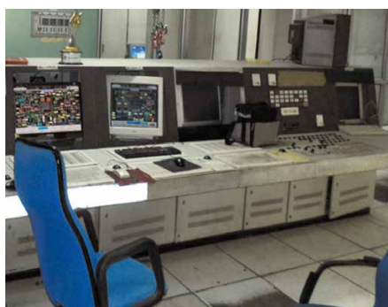
Before and after revamp photos of the central control room (CCR). The CCR layout was jointly designed by IOCL and Yokogawa India. The number of consoles was increased to improve efficiency.
