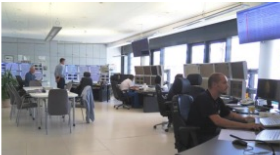
Evonik Oxeno Antwerp Control Room with 5 CENTUM operator centers featuring not less than 40 monitors for operators
