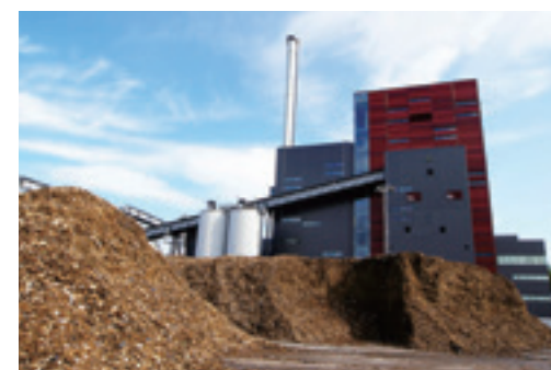
Biomass power plant
