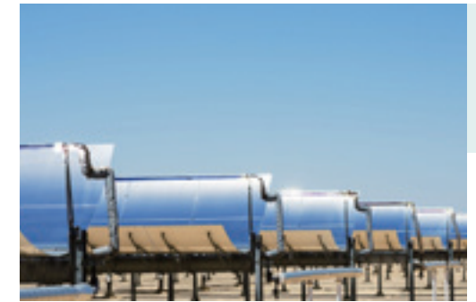
Solar thermal power plant
