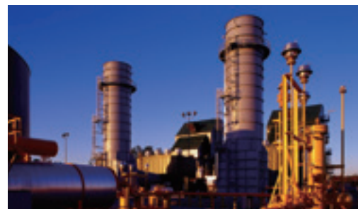
Combined cycle power plant
