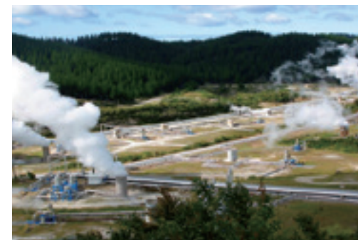
Geothermal power plant
