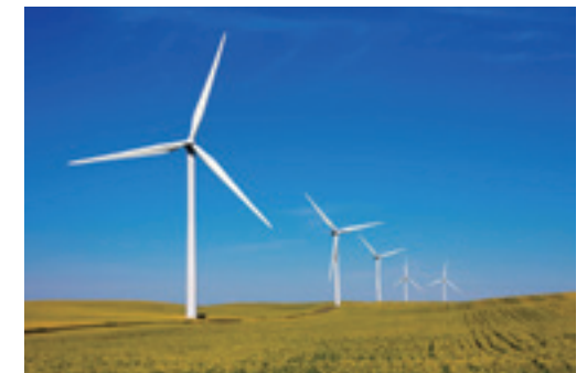
Wind power plant
