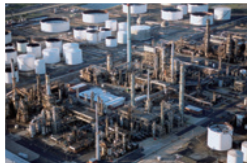
Industrial boiler plant/co-generation plant
