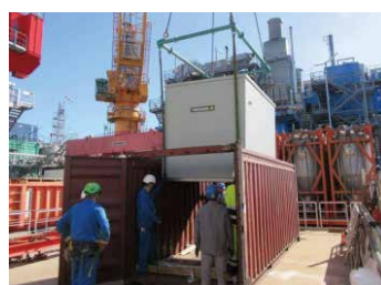
The analysis container being delivered on the Mittelplate
