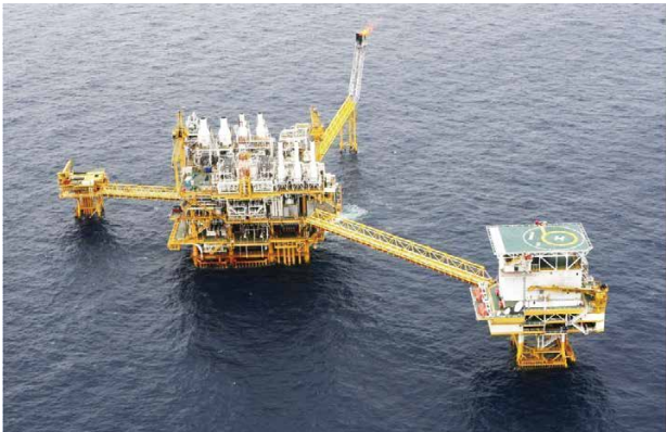
Central processing platform
