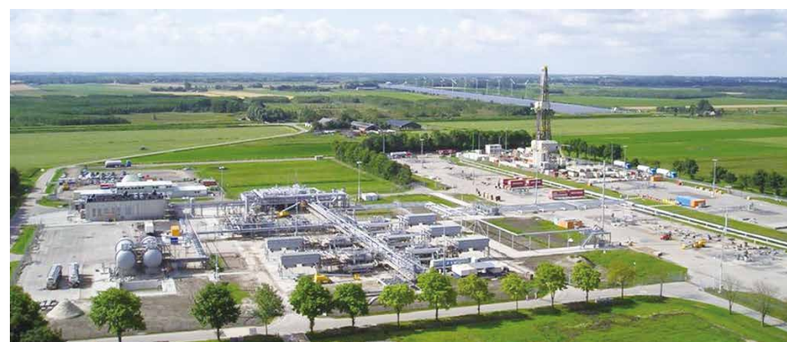
One of the 20 gas well clusters in Groningen province
