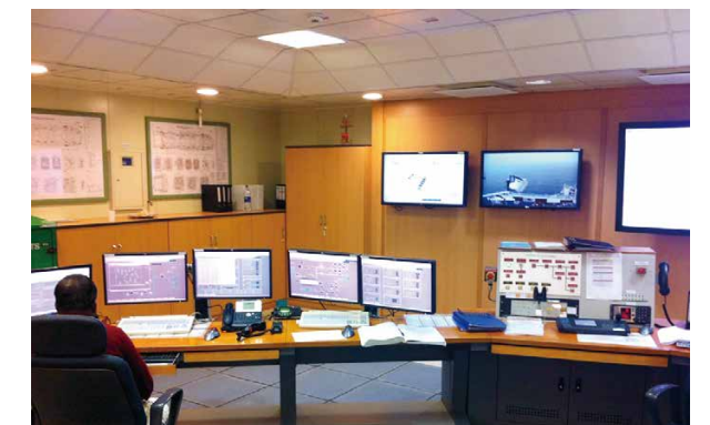
Control and monitoring of subsea and topside systems from the CCR aboard the Usan FPSO
