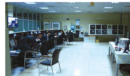
Pre-revamp CCR with legacy Honeywell TDC3000 system
