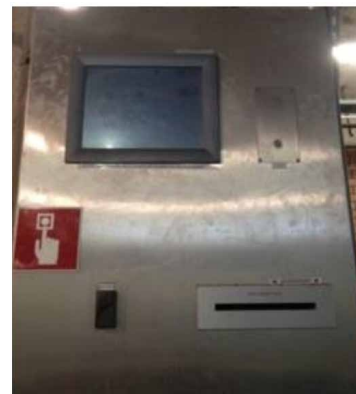
All bays are furnished with a loading panel equipped with a touch screen, intercom, barcode reader, card reader, and emergency button.
