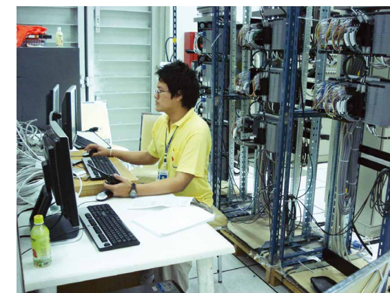
Field control station SAT in rack room
