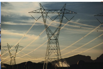
Temperature monitoring at power cable
