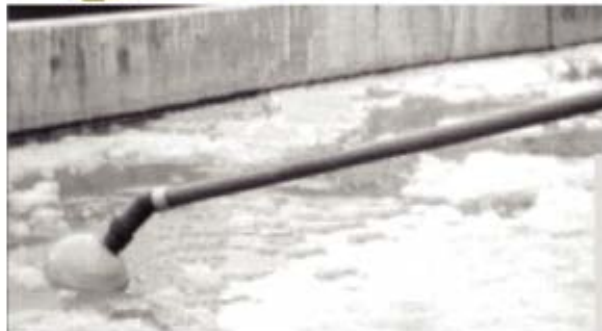
The sensor head is free from dirt even through a large amount of dirt floats on the surface of the sewage.
