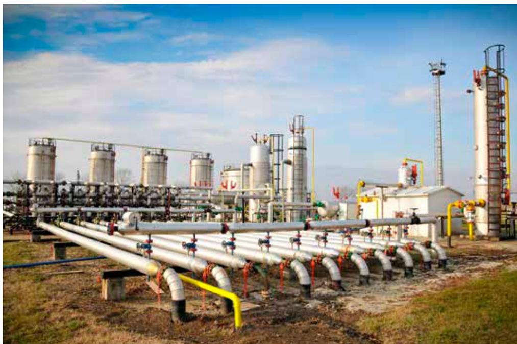
**Figure 1. Pneumatic controllers and mechanical pressure gages have no capability to communicate data from remote locations to a central control centre. Gathering information means a trip to the site.**
