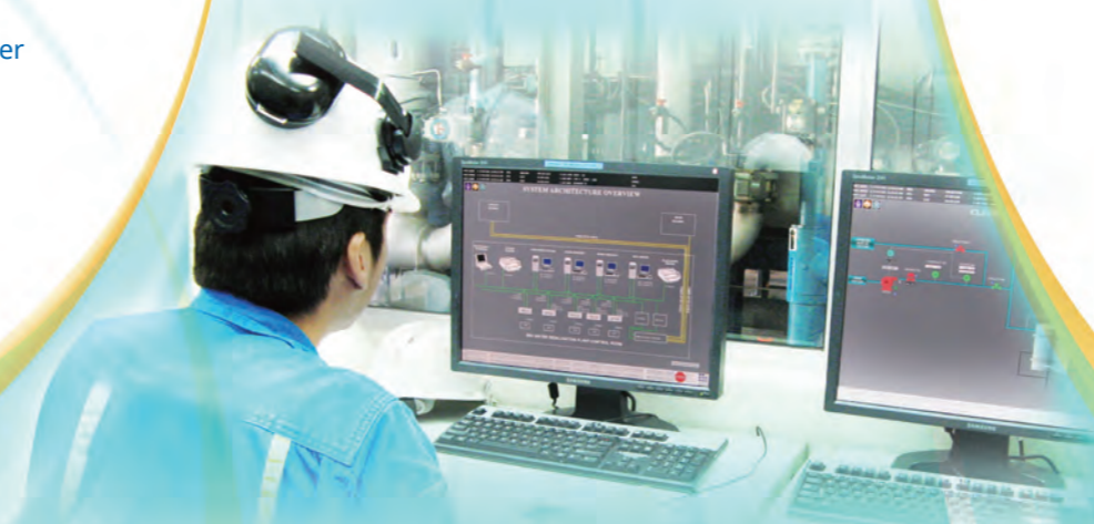
Main control room for field operations
