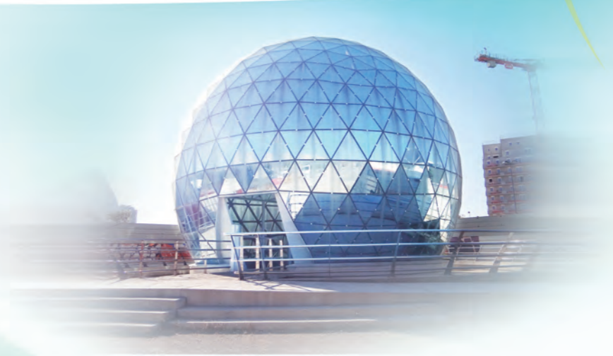
GEOLIDE wastewater purification plant in Marseille
