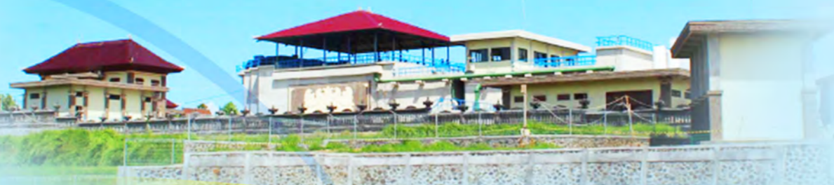
Petanu water treatment plant
