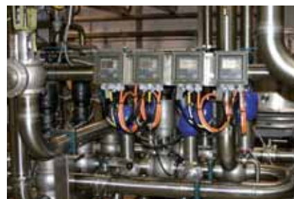
CIP is tightly controlled with Yokogawa's Inductive Conductivity Systems
