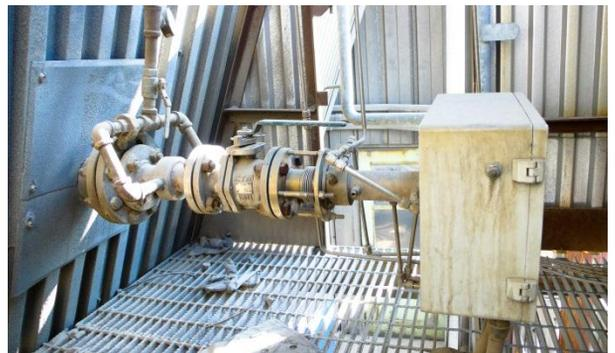
The TDLS launch unit is located outside and is exposed to a wide range of weather conditions.
