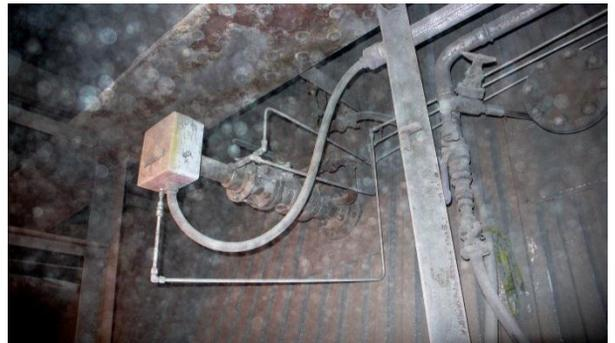
The TDLS detect unit in a fly ash-filled environment. It is noticeably covered with ash.
