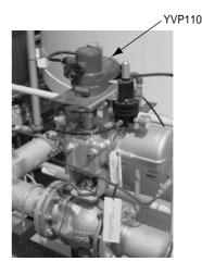
**Figure 1** YVP110 Installed in Actual Plant (by courtesy of the Fushiki plant of Nippon Paper Industries)
