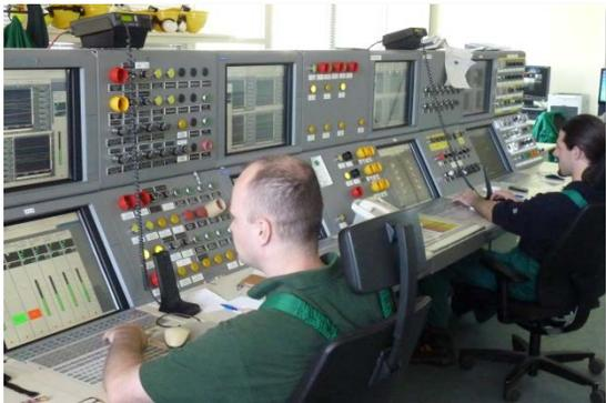
Picture 4. Unit operators in front of Yokogawa CS3000 HMI in CCR unit
