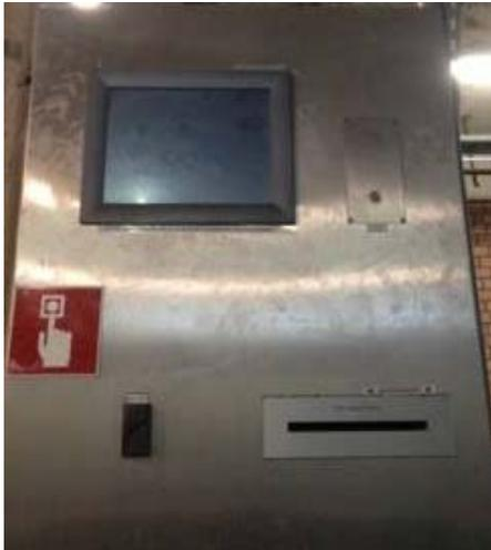
All bays are furnished with a loading panel which is equipped with a touchscreen, intercom, barcode reader, card reader and emergency button.
