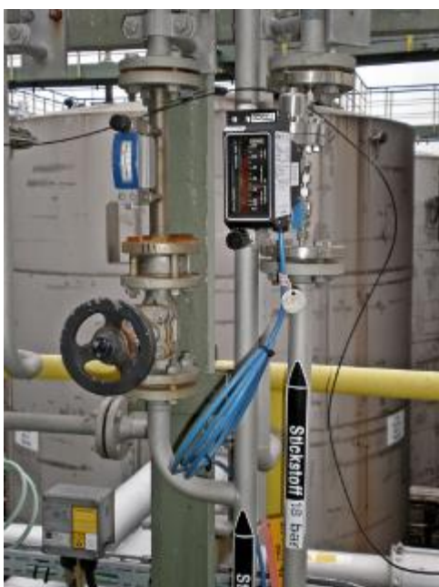
Fig. 6 New measurement point (right) for the nitrogen flow into the main column
