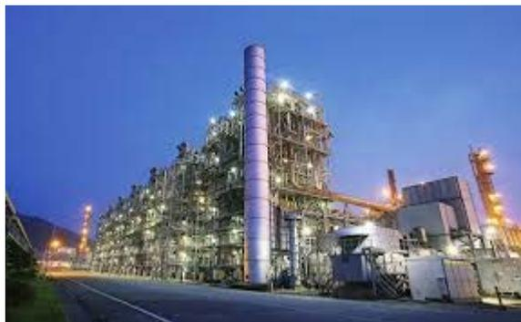
All of the processes at this ethylene plant are controlled by a Yokogawa CENTUM CS3000 production control system that was engineered, installed, and commissioned by Yokogawa Korea. To further enhance operations at this plant, Yokogawa Korea introduced the Exapilot operation efficiency improvement package in 2006.
